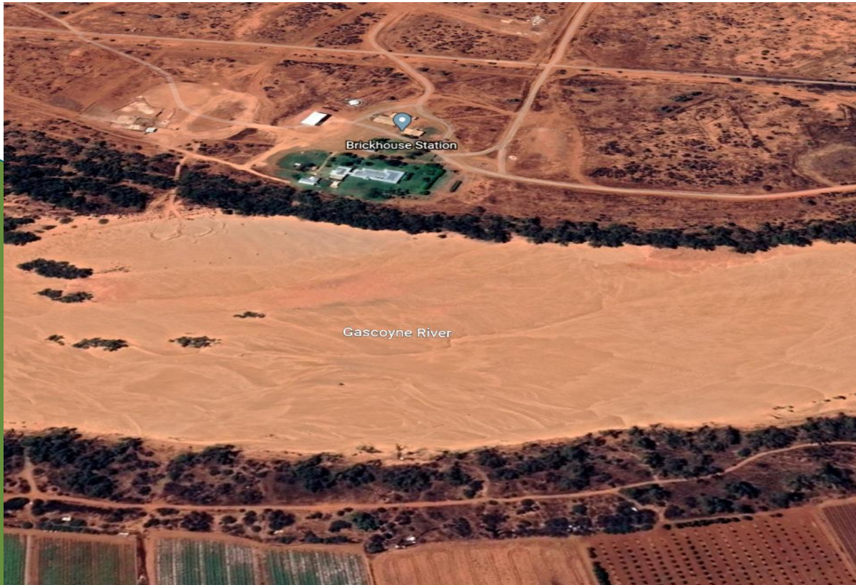
Figure 24 Brickhouse Station (Google Earth)
