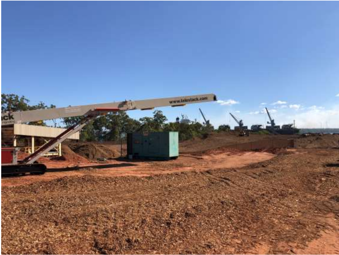
Woodchip processing and ship loading facilities, Tiwi Islands (Melville Island), NT
