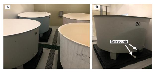
**Figure 8.** (A) Four 5,000 L tanks in larval rearing room and (B) close up of one 5,000 L larval rearing tank, showing two 50 mm tank outlets.
