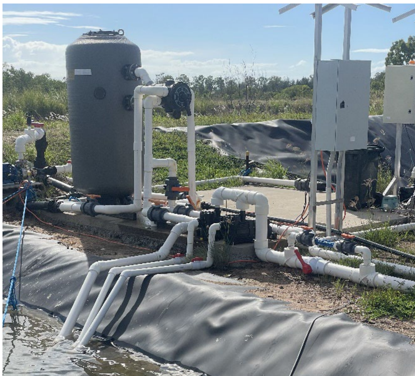
Figure 4. Infrastructure connected to two pumps required to support water flow in enclosures used for TRL grow-out.
